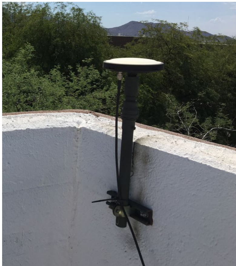
Figure 2-5: Roof mounted antenna
